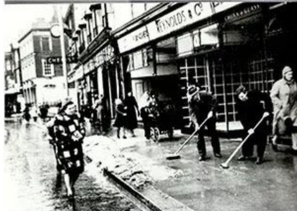
Volunteers clear up glass and debris after an air raid
